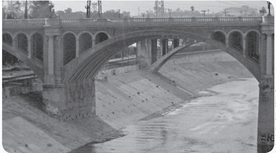
Los Angeles River Bridge B&W by Downtowngal
